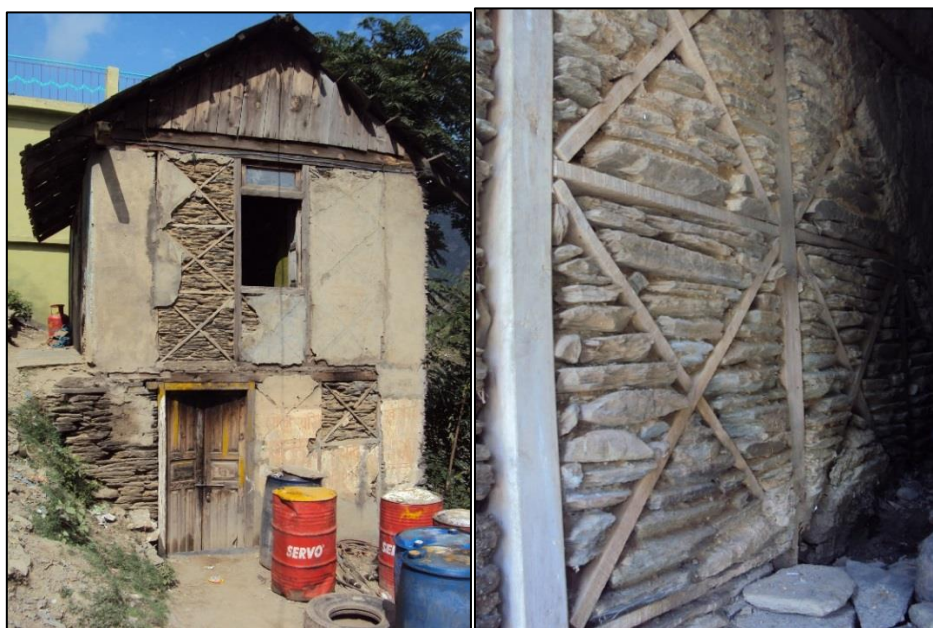
Figure 19: Dhajji Dewari Type House (Shimla, 13 th November 2013)
