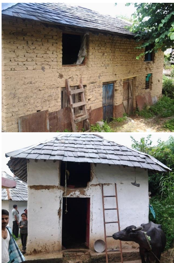
Figure 58: Cowsheds made of unburnt brick/mud wall and slate roof
