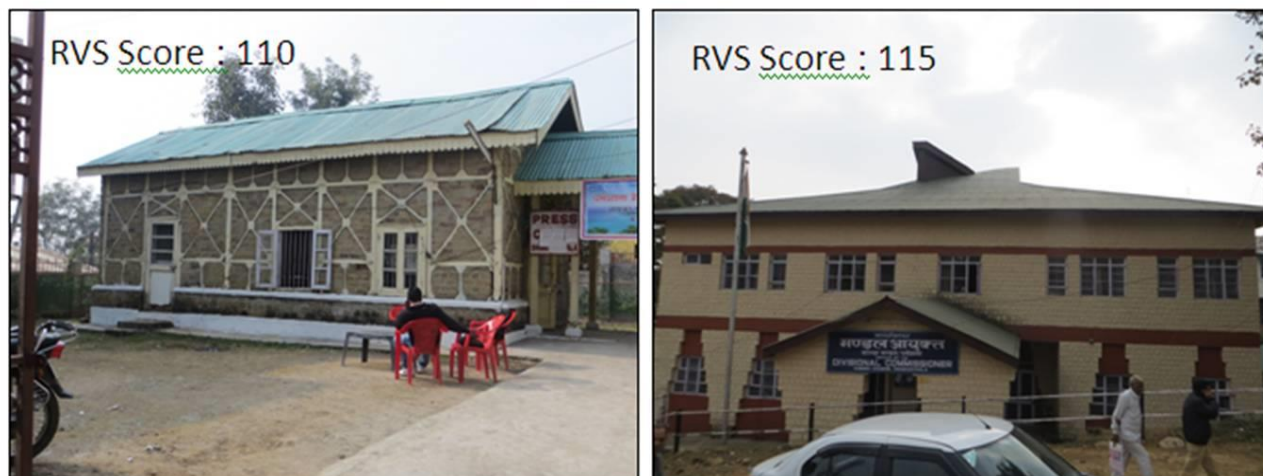
Figure 88: General View of stone masonry Buildings
