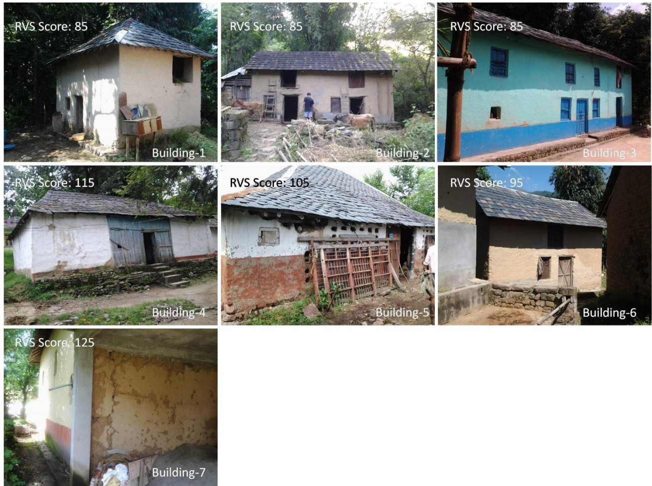
Figure 89: General View of rammed earth Buildings
