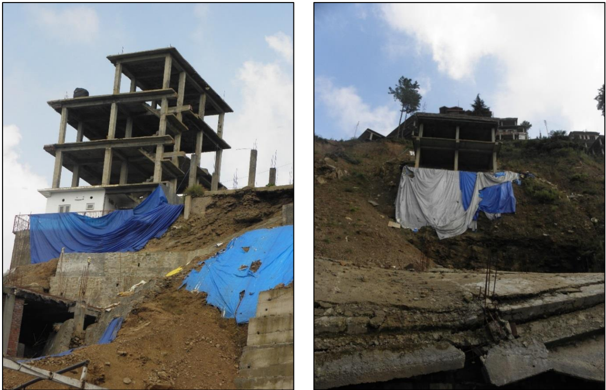
Figure 30: Construction of building on sloping site
