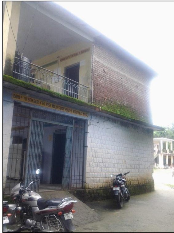
Figure 25: Hybrid Construction (Stone masonry and brick masonry)
